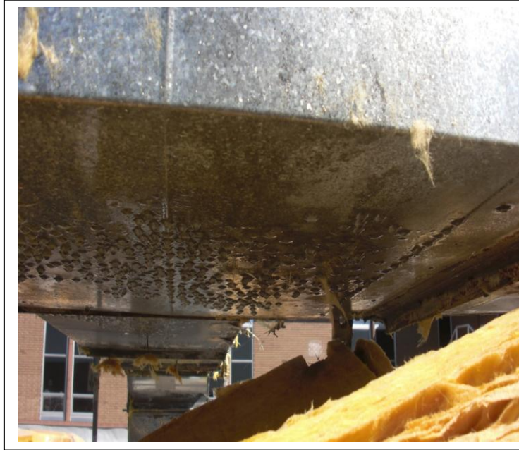
Heavy condensation droplets
