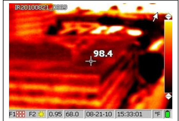
Metal drain cover
