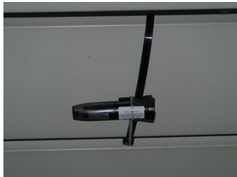
Typical Data Logger installation
